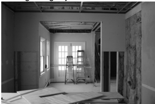
beginning drywall installation
