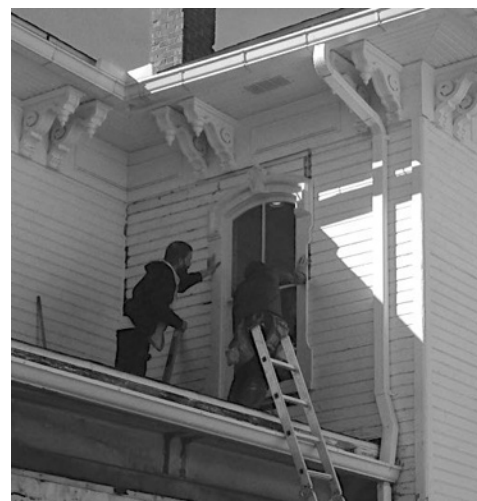
New Window Installation
